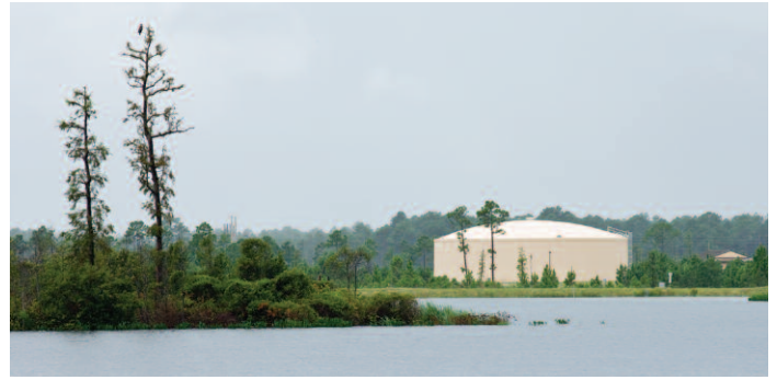
A reservoir holds reclaimed water prior to it being pumped into a storage tank in Port Orange.
